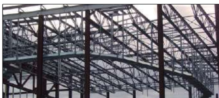
Roofing and Cladding
