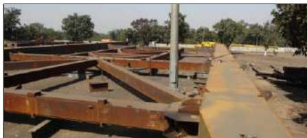
Fabrication and Erection
